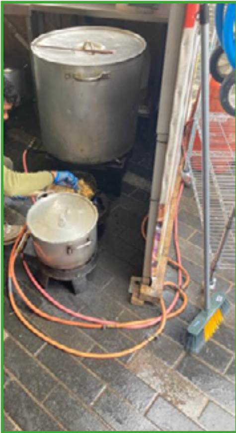
Incorrect use of excessive length of flexible orange hoses, connected with jubilee clips.
